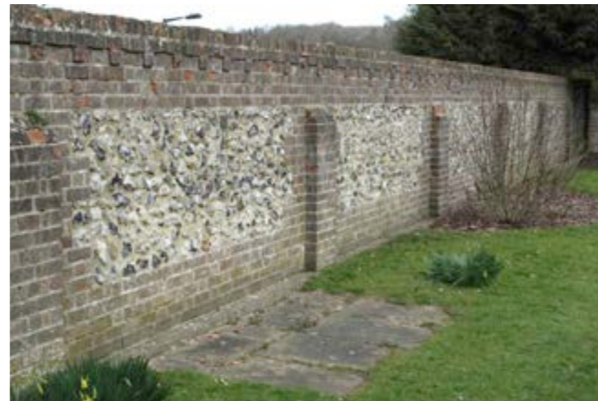
Plate 4.26: Section of wall showing flint panels
